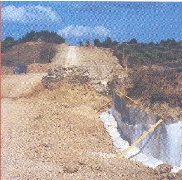
Figure 5. Preservation of top soil with geotextile in ecologically sensitive areas.
